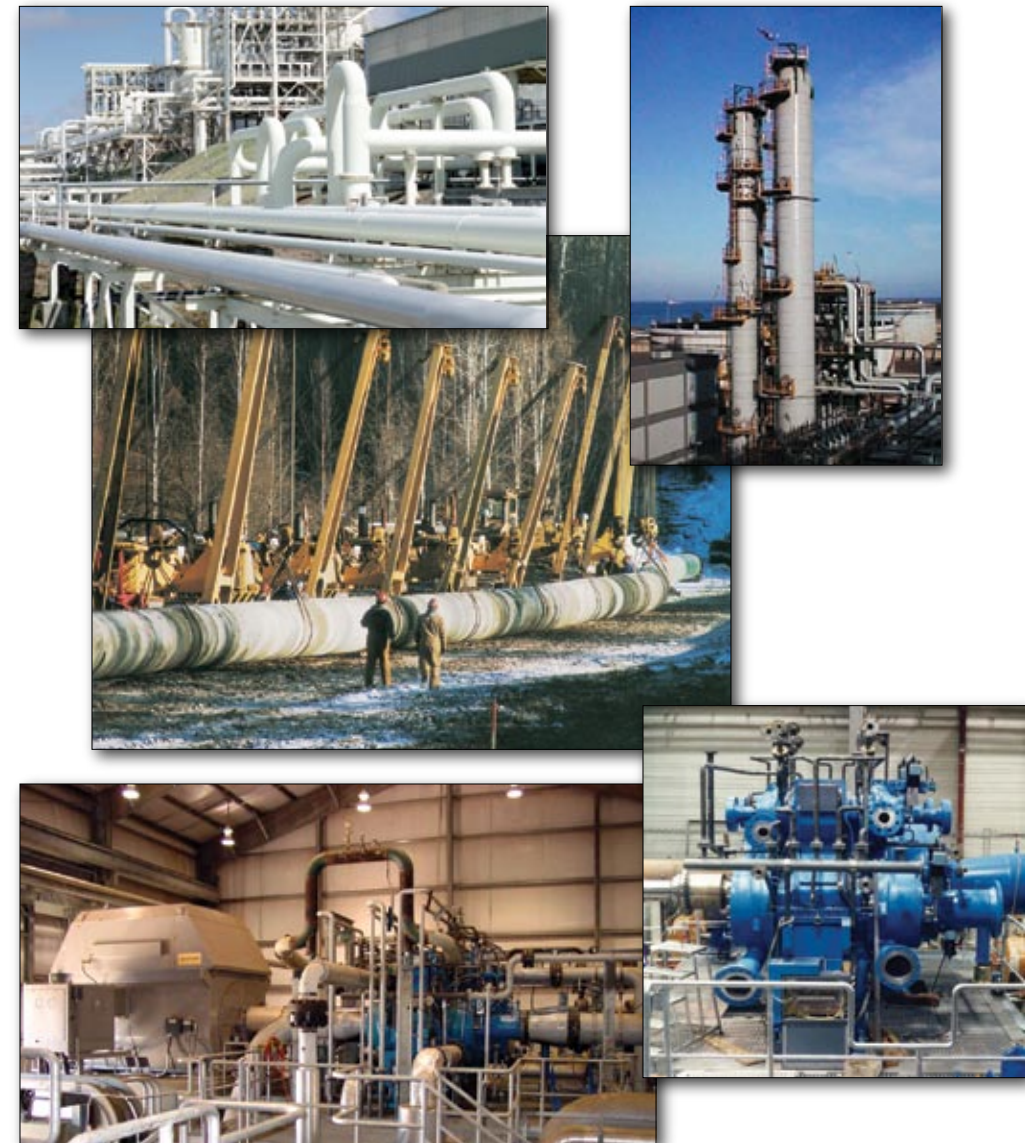
Top left and center: In the future, a more extensive CO 2 pipeline network will probably be constructed. Top right: Selexol™ towers at a recent integrated gasification combined-cycle start-up. Bottom: CO 2 compressors at the Dakota Gasification Company's synfuels plant in central North Dakota each move about 55 million cubic feet of CO 2 a day at a discharge pressure of 2700 psi.
