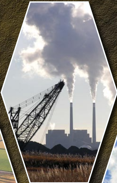
Coal-Fired Power Plant
