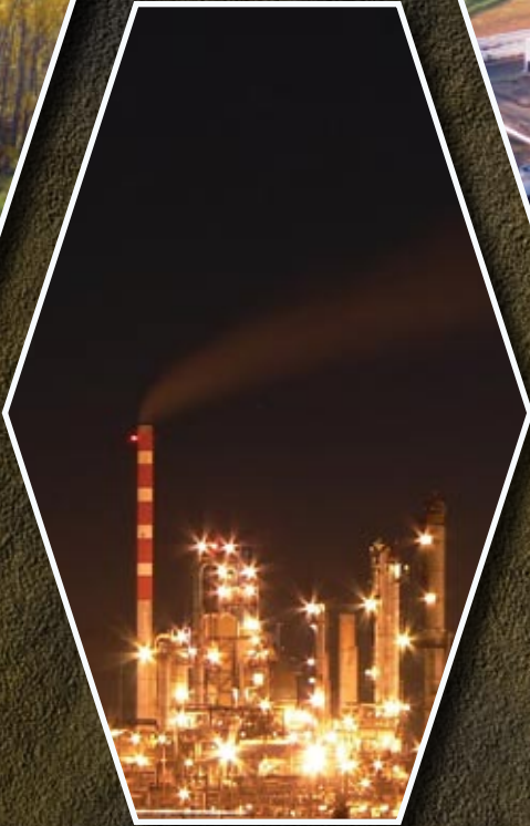
Gas Processing Plant
