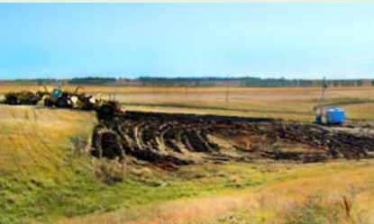
Reclamation of the site began with earthmoving to reestablish the surface contour. Site reclamation was deemed successful after two summers, with vegetation well-established and suitable for grazing.
