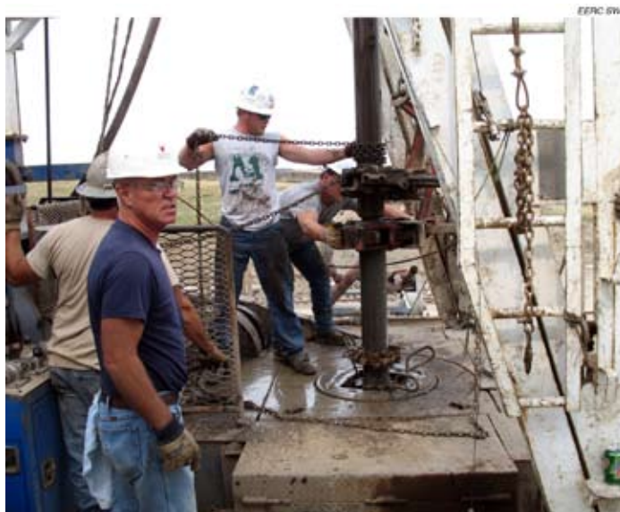
Figure 2. Drilling a well at the Lignite Field Validation Test Site.
