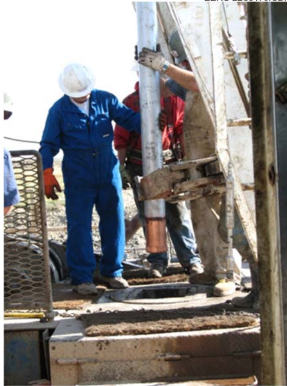
Figure 3. Core barrel.
