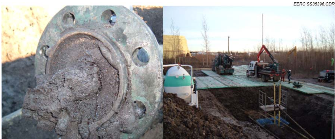
Figure 15. Operation to clear a plugged flowline.
