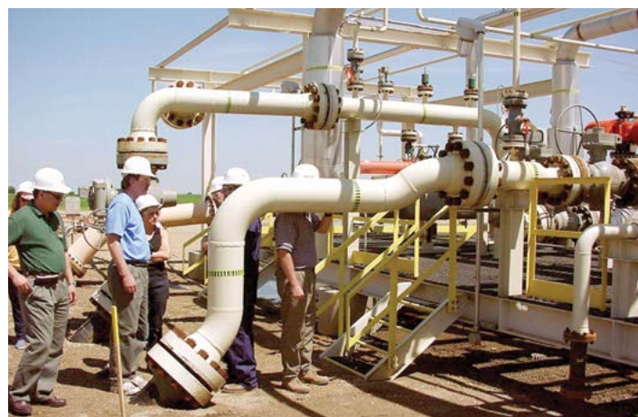
Figure 2. CO 2 is pumped 4800 feet underground at the CO 2 injection site in the Weyburn–Midale Field in Saskatchewan, Canada.
