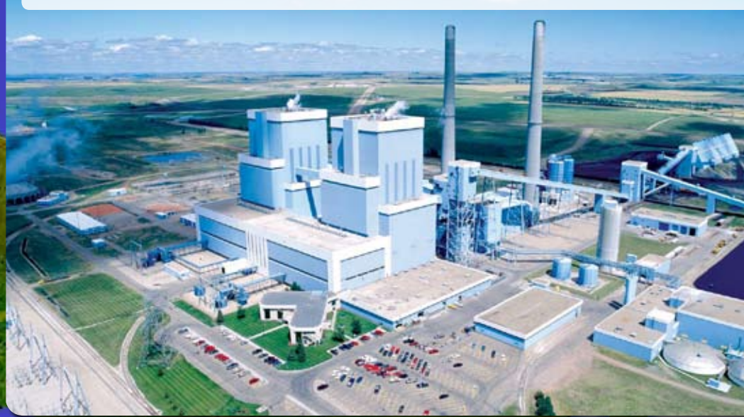
Basin Electric Power Cooperative's Antelope Valley Station is a pulverized coal-fired power plant.
