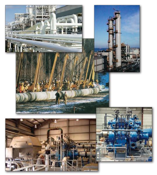
Top left and center: In the future, a more extensive  $CO_2$  pipeline network will probably be constructed. Top right: Selextol<sup>TM</sup> towers at a recent integrated gasification combined-cycle start-up. Bottom:  $CO_2$  compressors at the Dakota Gasification Company's synfuels plant in central North Dakota each move about 55 million cubic feet of  $CO_2$  a day at a discharge pressure of 2700 psi.
