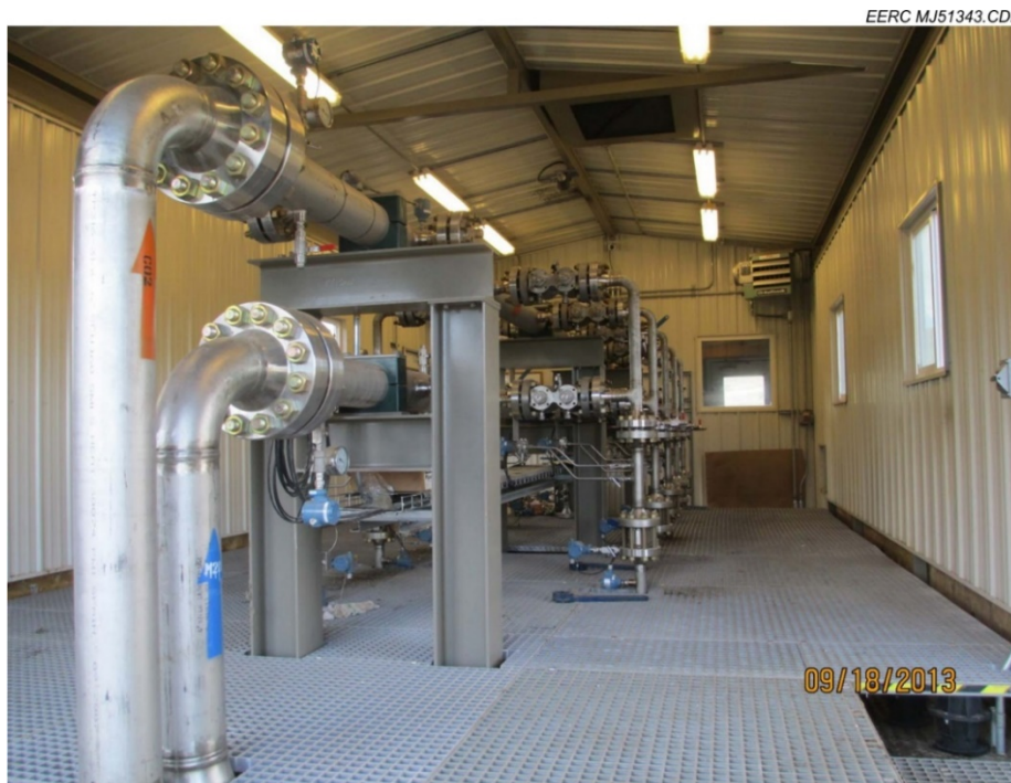
Figure 12. An injection manifold at Bell Creek (taken from Rawson, 2014).
