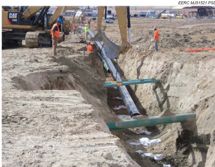
Figure 6. Greencore pipeline construction with pipe in trench (taken from Blincow, 2013).
