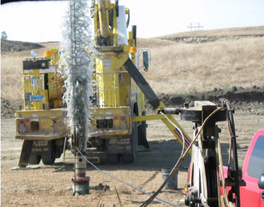
Figure 3. Perforation job on a well at the lignite field site.
