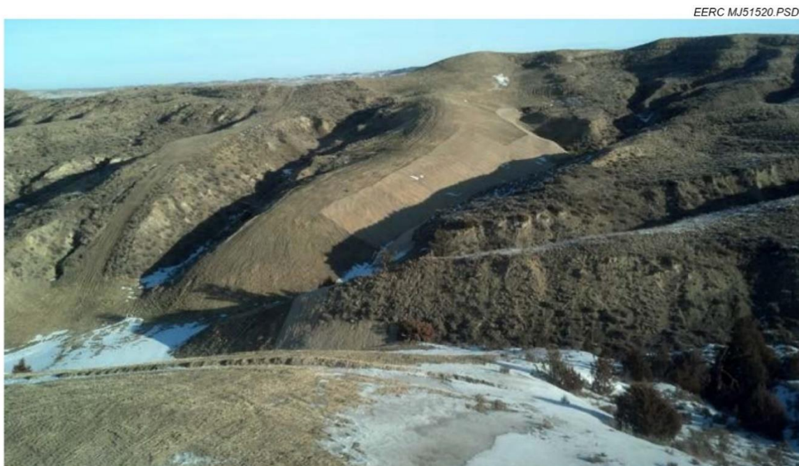
Figure 12. Photograph of Greencore pipeline route through a hilly area taken postreclamation (taken from Blineow, 2013).
