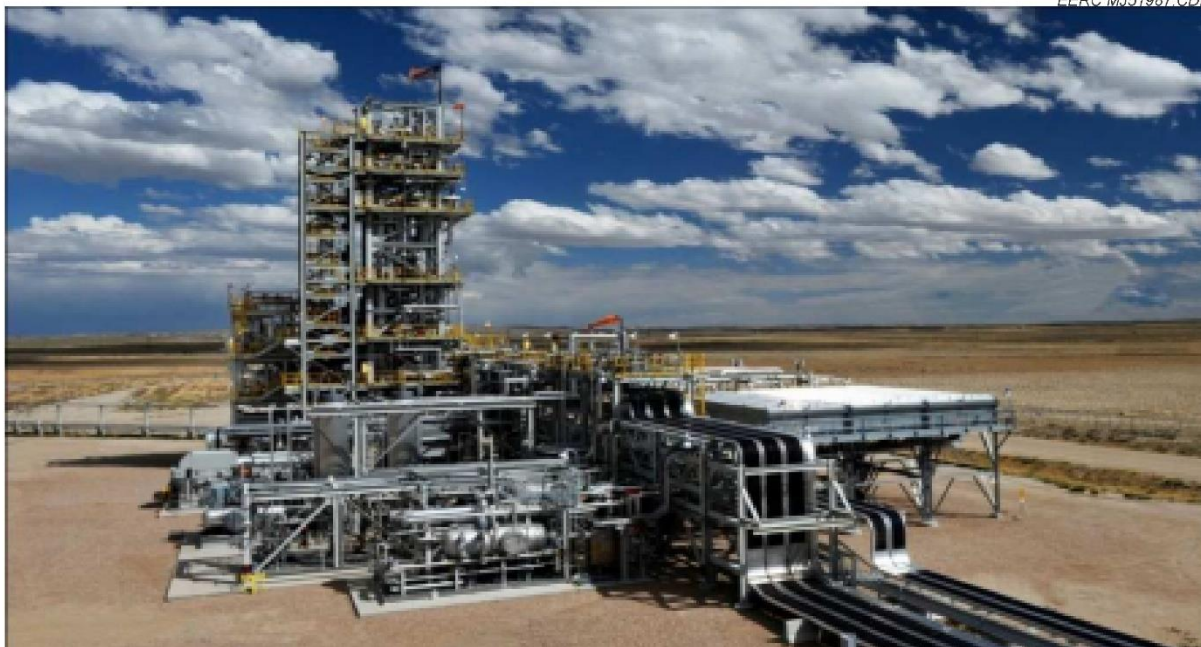
Figure 6. Photograph of the CFZ™ demonstration unit at the Shute Creek Gas-Processing Facility (taken from Khayyal, 2013).
