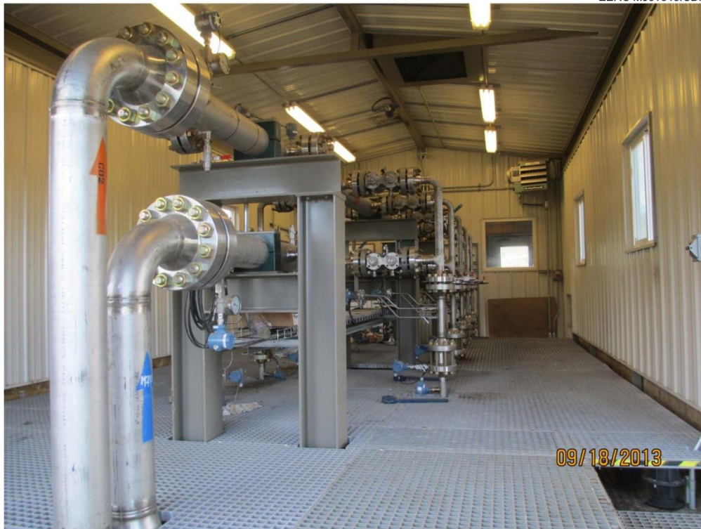
Figure 20. An injection manifold at Bell Creek (taken from Rawson, 2014).
