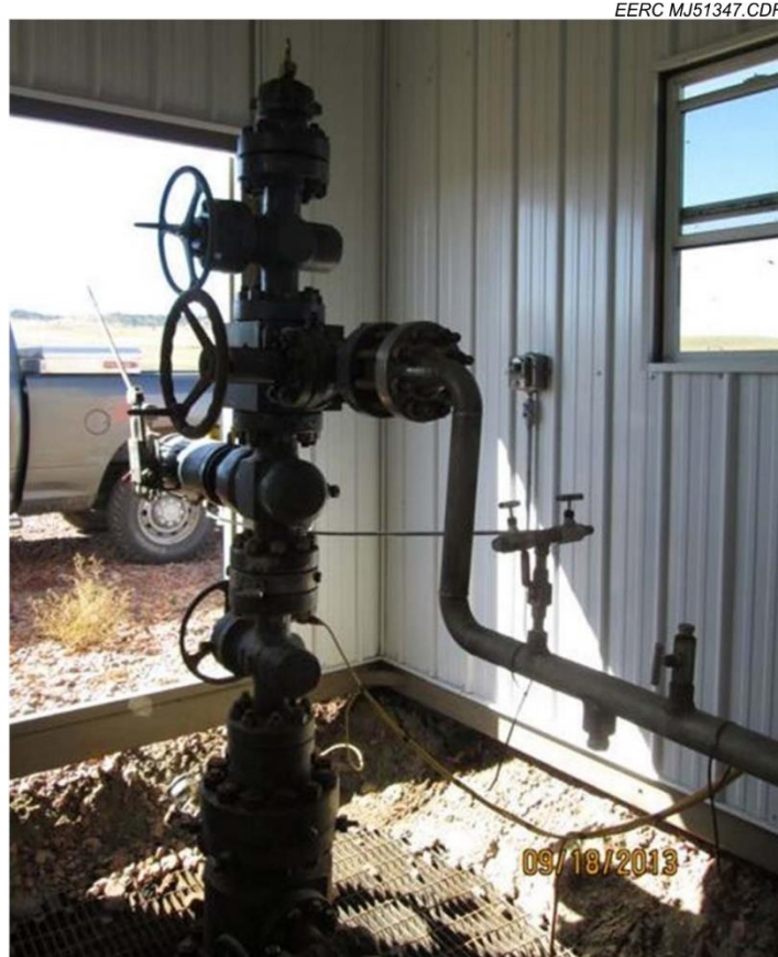
Figure 24. CO 2 or water injector wellhead (taken from Rawson, 2014).
