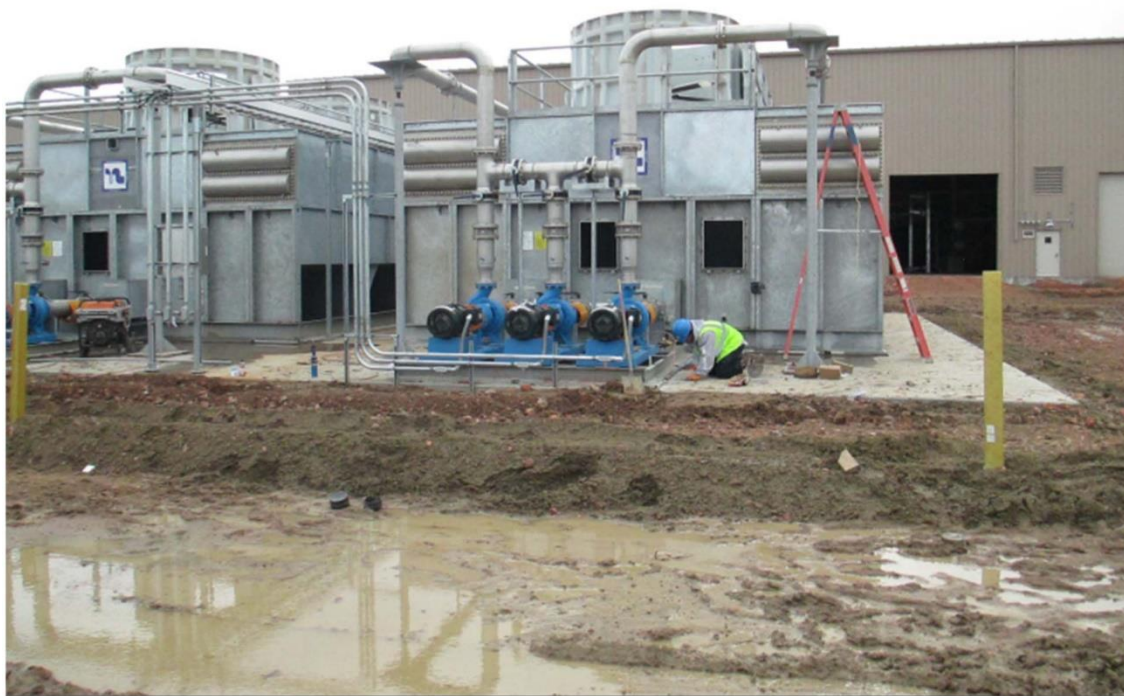
Figure 22. Bell Creek heat media system during its construction (taken from Walsh and others, 2013).
