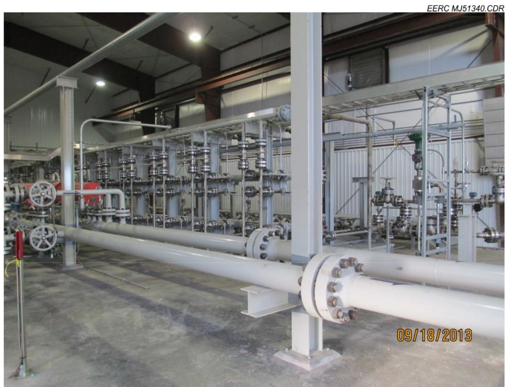
Figure 17. Bell Creek test site production manifold (taken from Rawson, 2014).
