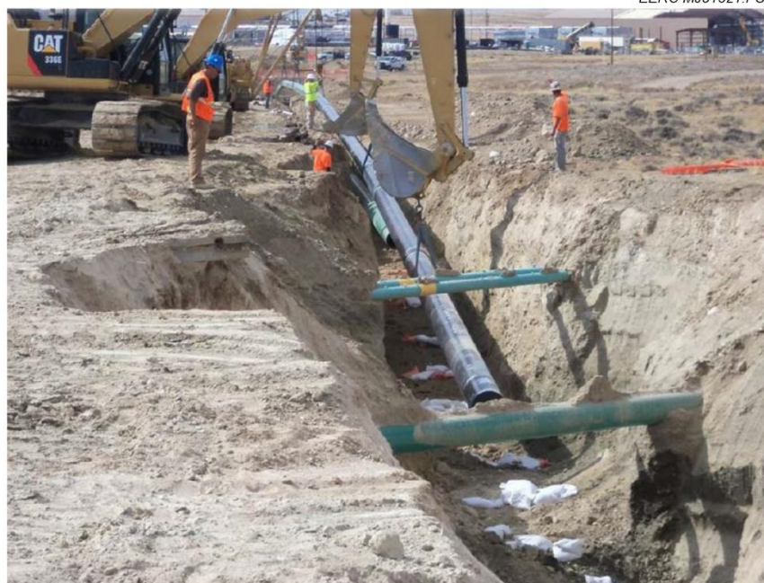
Figure 14. Greencore pipeline construction with pipe in trench (taken from Blincow, 2013).
