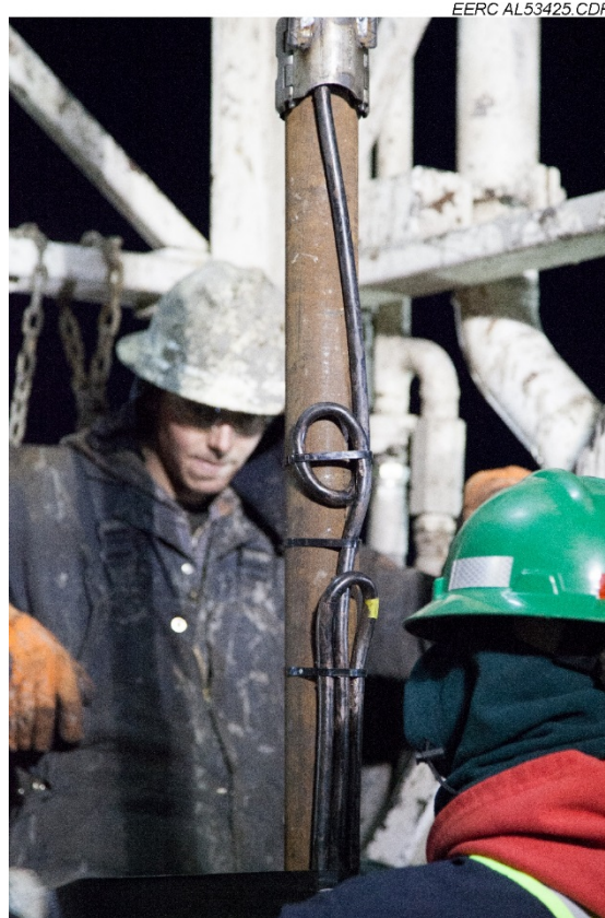
Figure A-7. Photo of secured array cables along the casing.
